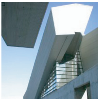
This is a nice detail, showing the contrast between solid and glazing. There is a strong channel-groove underneath. Below, we also see that doorways are cut into the volumes.
